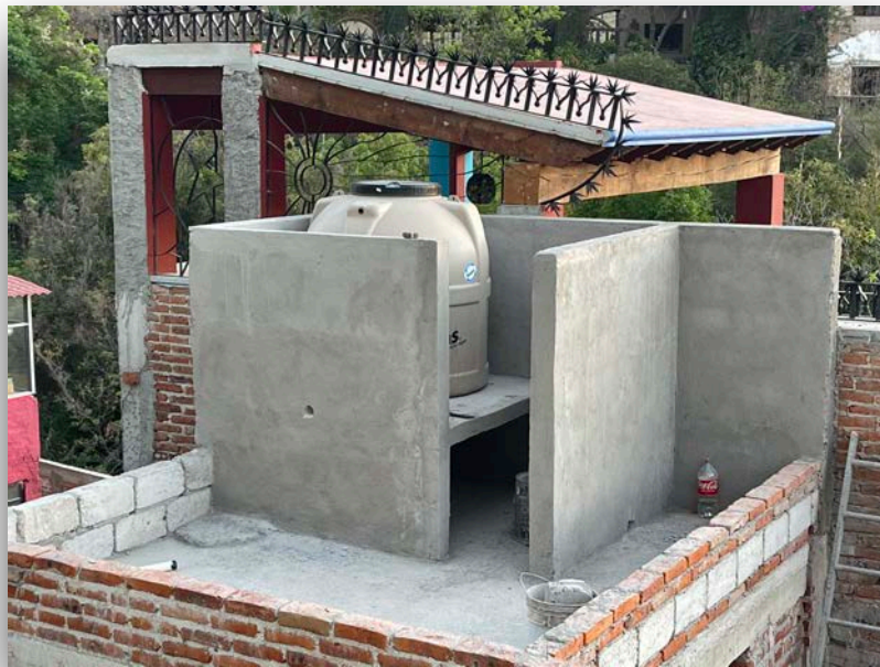
Indeed, a water tank is inside the little square addition.
